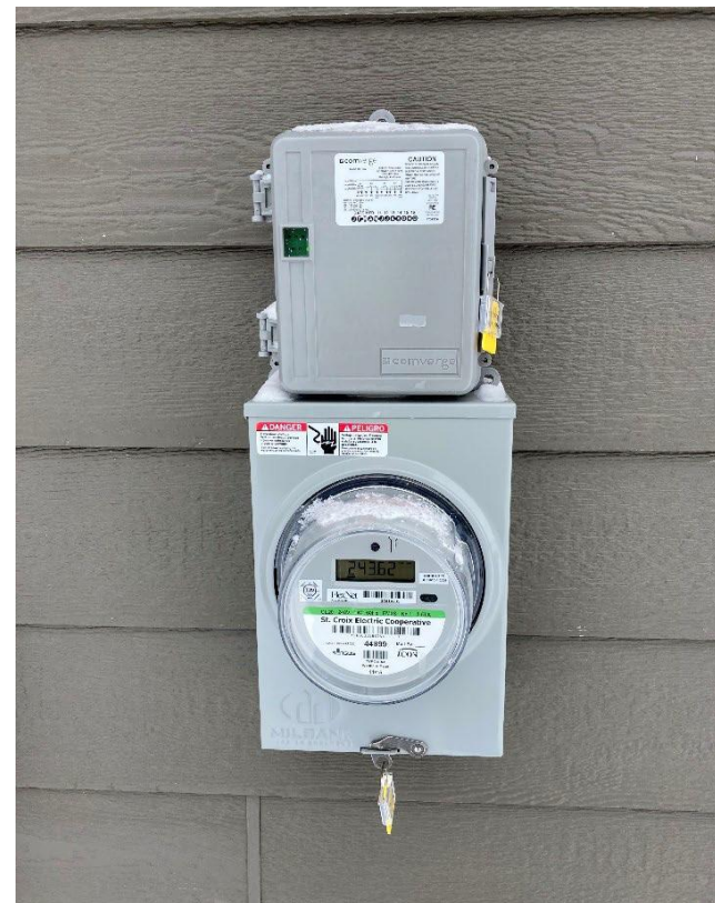
Example of off-peak installation – meter supplied by SCEC
